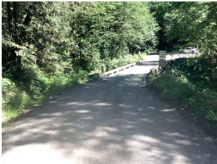
Approach from Right Bank when facing downstream
