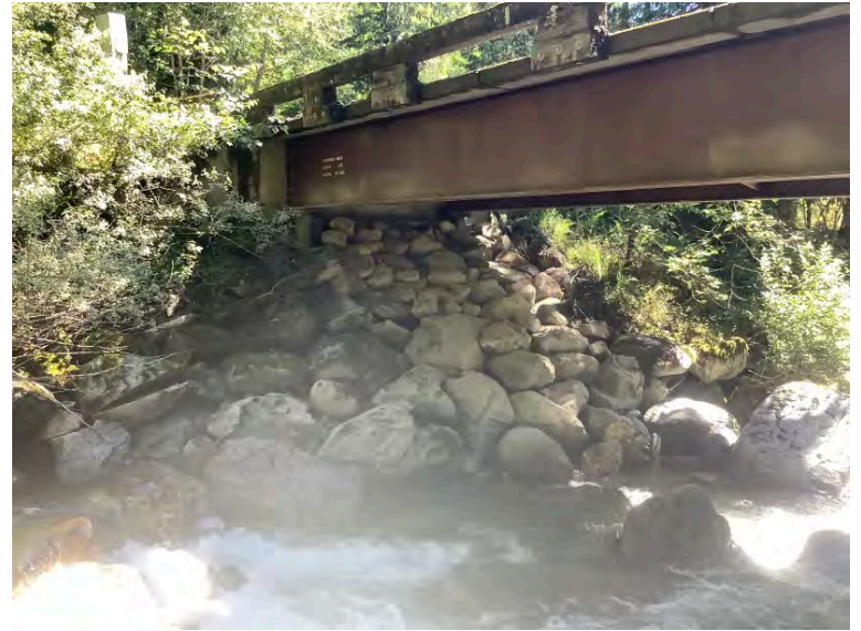
Left Bank Abutment when facing downstream
