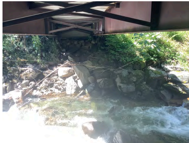
Right Bank Abutment when facing downstream
